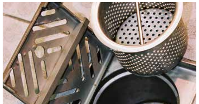
You must have bucket traps in sink and floor drains in commercial kitchens.
