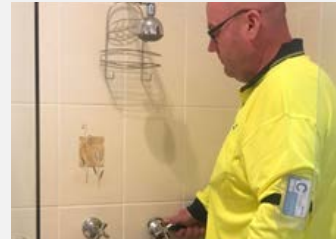
WaterFix® plumber repairing an indoor tap leak
