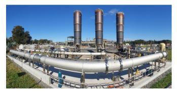
Figure 3 Waste Gas Burner Pipework Upgrades
