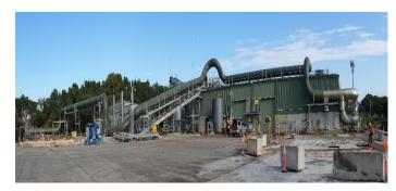
Figure 2 Installed ventilation ductwork on biosolids building and area where biofilter previously was
