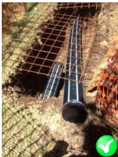
Figure 1 Pipes capped overnight in trench
