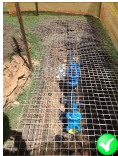
Figure 2 Fittings capped overnight in trench
