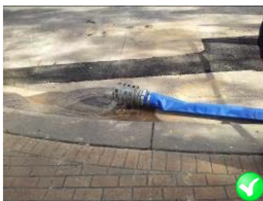
Figure 8 Discharged water directed away from trench
